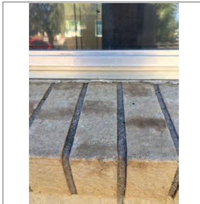
Caulking is dried around windows. Replace
