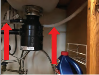
Dishwasher drain is not high looped
