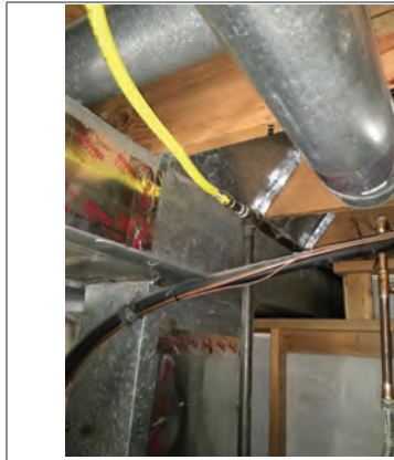
CSST tubing may not be properly bonded
