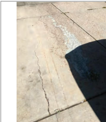
Driveway. Note: spalling and typical cracks
