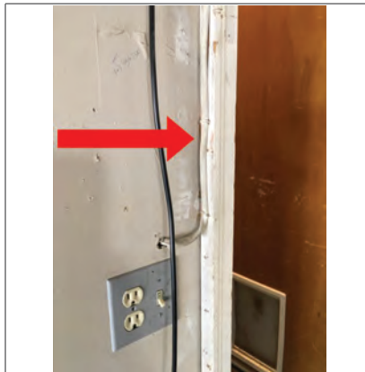
Electrical wiring not in conduit
