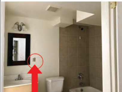
Basement bathroom Receptacle cover plate is missing
