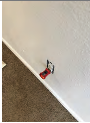
Loose receptacle and missing cover plate
