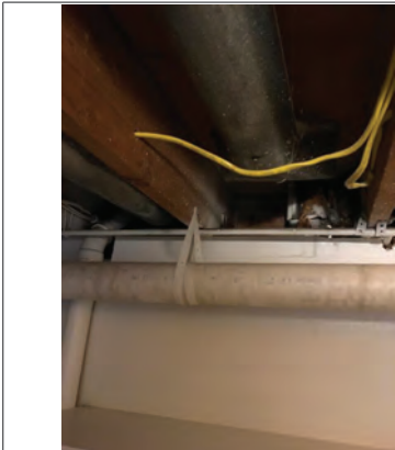
Insulation is missing on rim joists
