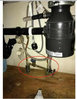
Corrosion present. Monitor for leaks.
