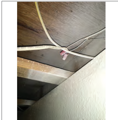
Spliced wires not in junction box
