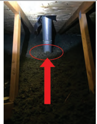
Furnace and water heater exhaust vent in contact with insulation. Create void space with shroud.
