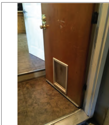
Door leading to home is not a fire door
