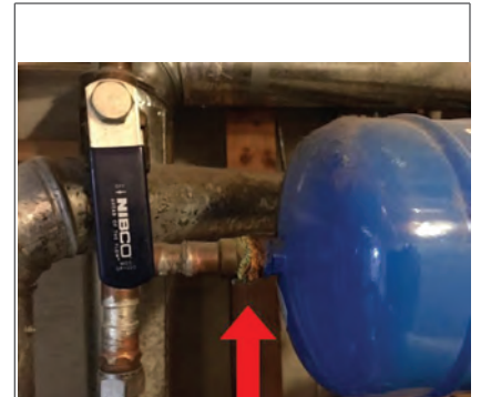
Corrosion at expansion tank
