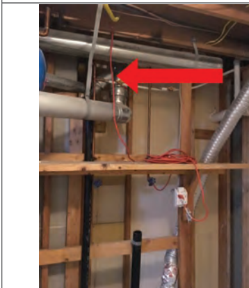
Extension cord to stove. No GFCI in basement
