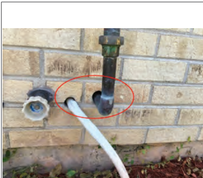
Recommend caulking around wall penetrations
