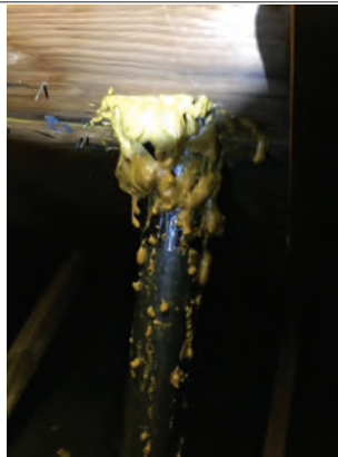
Unprofessional exhaust fan insulation.
