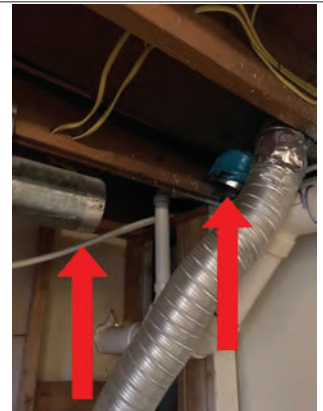
Combustion air venting not connected
