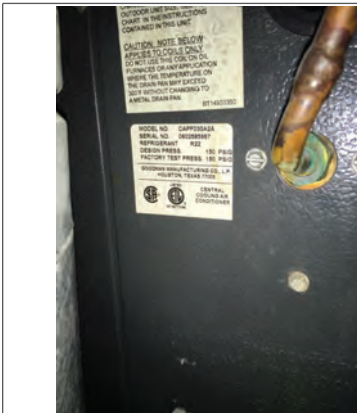
House air conditioning evaporator coil data plate
