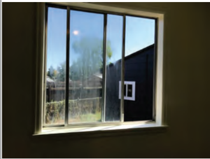
Window has evidence of leaking gas
