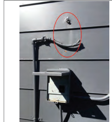
Condensate line is disconnected
